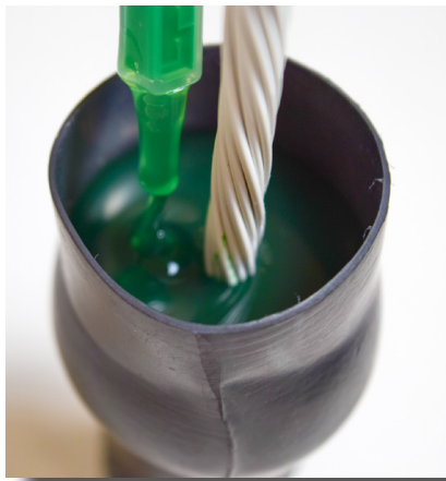
Self-Leveling Green® being injected to connector boot.
