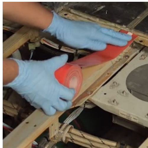
HI-TAK Polyurethane Rolled Sealant (PRS) Installation
