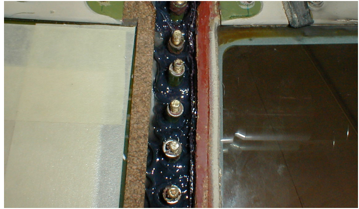
Thixflex Black® installed in panel to create water tight seal
