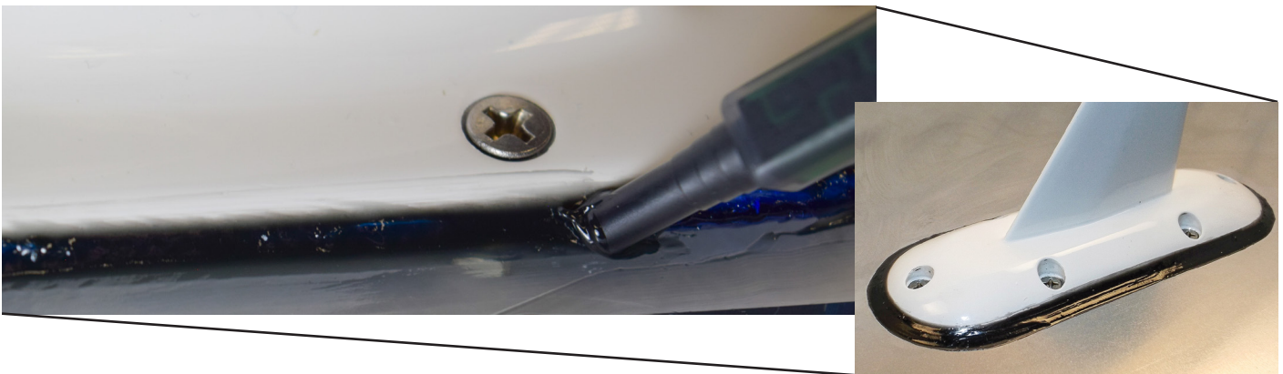
Thixoflex Black® applied as a quick-cure fillet seal
