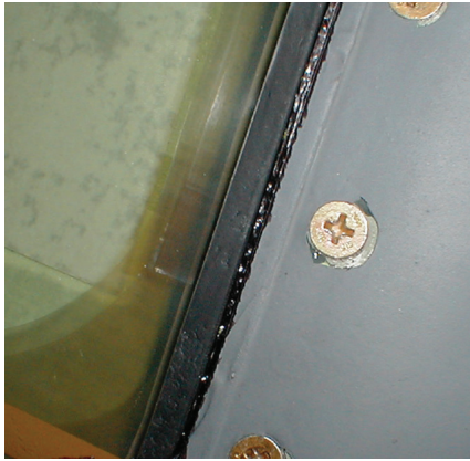
Thixflex Black® injected around cock pit windows
